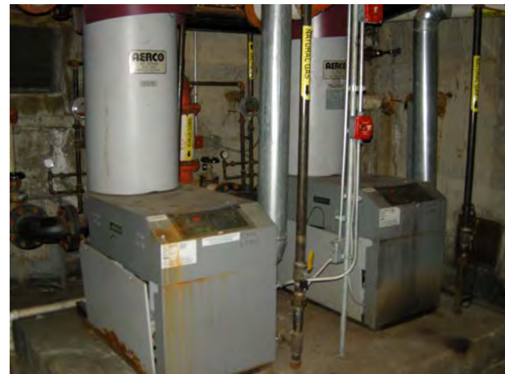
One of seven heating/domestic hot water plants.
