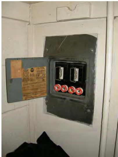
Typical dwelling unit 60-Amp fuse box to be upgraded to 100-Amp circuit breaker panel
