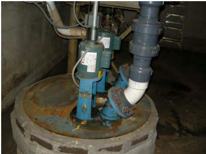
One of seven storm water pump stations
