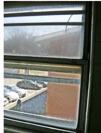
Typical interior window showing inefficient interior storm window.
