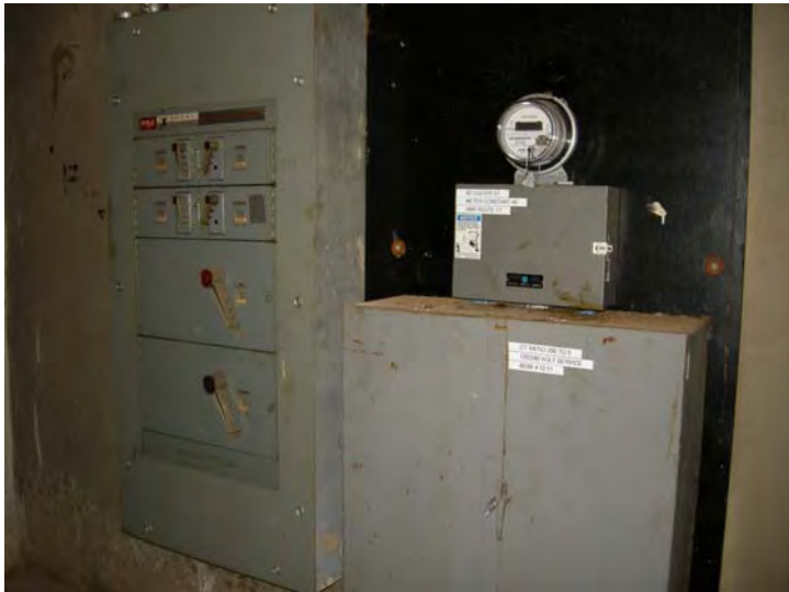
Typical electrical service distribution buss to be upgraded
