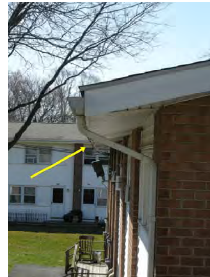
Building soffits are sagging badly throughout the development
