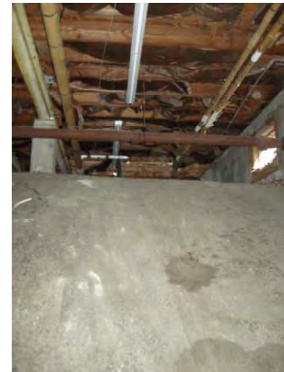
Typical un-insulated crawl space
