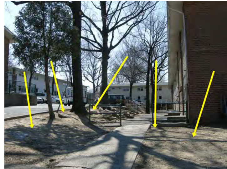
Examples of the typical site erosion observed throughout the site
