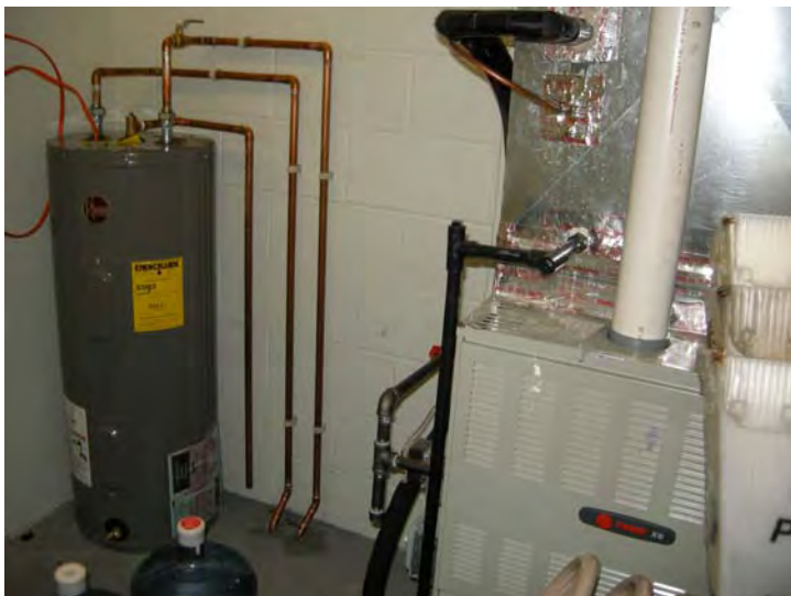
Heating/cooling and domestic hot water system at the community building
