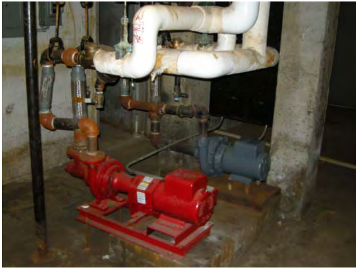
Typical hydronic heat circulation pump stations
