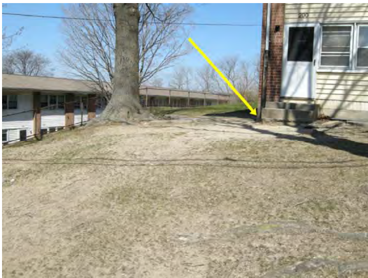
Erosion at base of entry stairway
