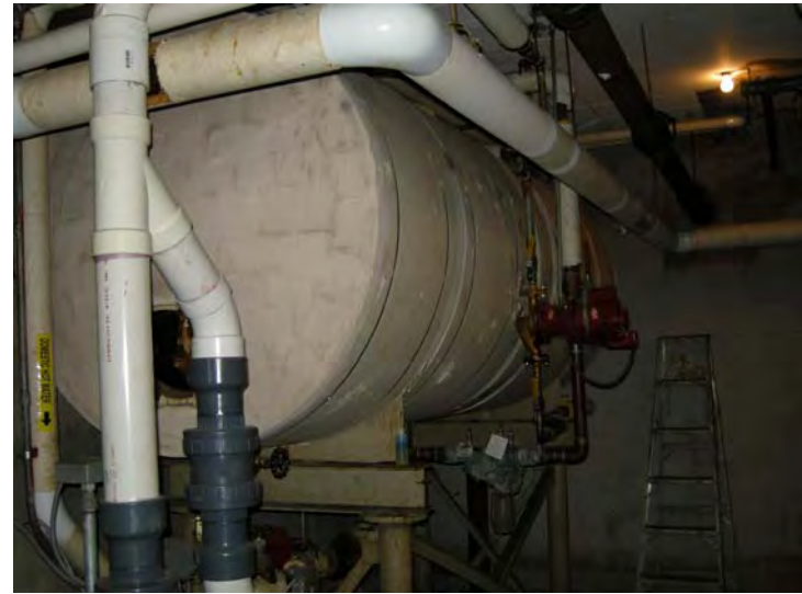
One of seven DHW storage tanks.
