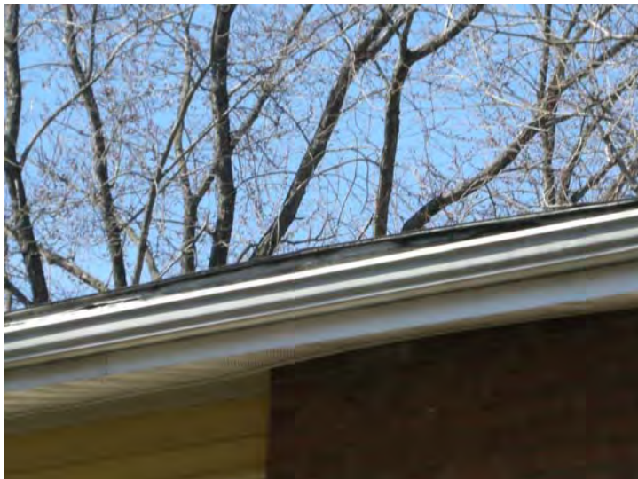
Close up of sagging soffit section
